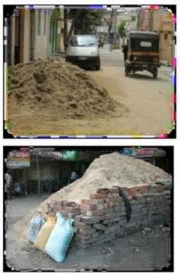
(Sand should not be left without enclosure, as the sand spills on the road, causing risk of skidding to 2-wheelers)
